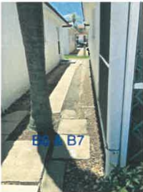
Unrestored P.R. Excavation - B7
